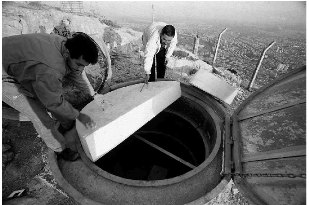
Figure 4. Installing thermal cover in a seismic vault. In climates with big diurnal temperature changes the cover should be positioned lower in the vault where external ground temperature doesn't change significantly.
