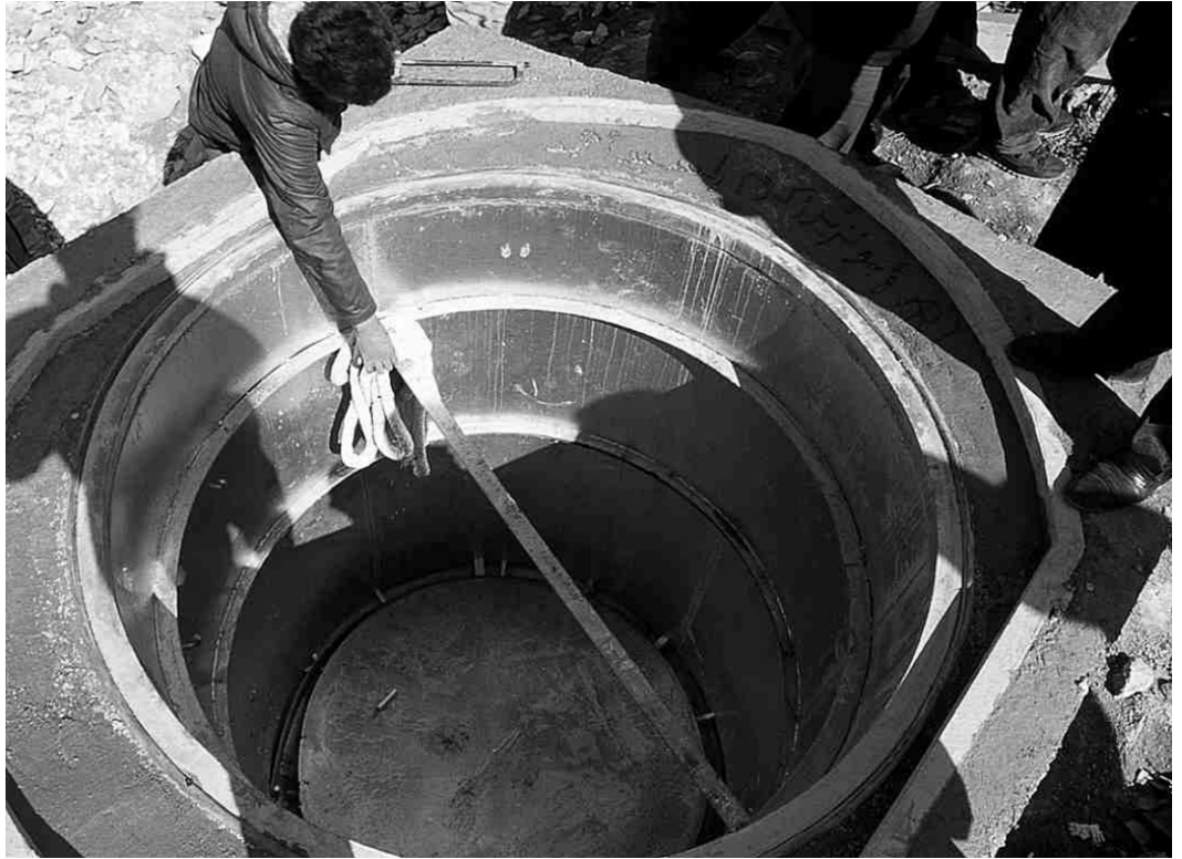
Figure 2. Interior of a seismic vault made of welded metal sheets. The vault is big enough to accept weak and strong motion instrumentation as well as data acquisition and transmission equipment.
